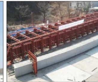
Curved Box Girder 품조립
