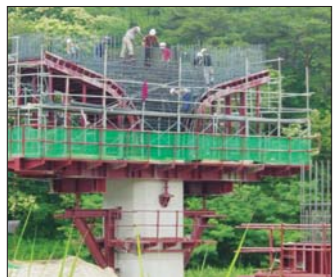
Side Panel Open 철근작업
