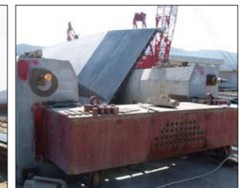
Pretension Beam 품조립
