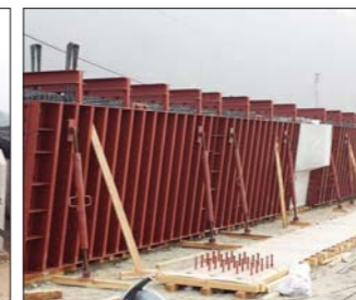
PDF Girder 품조립
