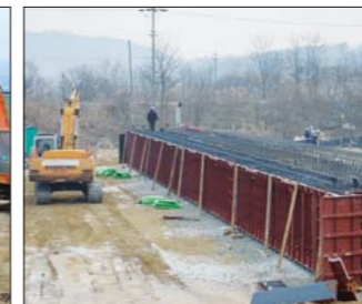
EX-B.I.B Girder 품조립
